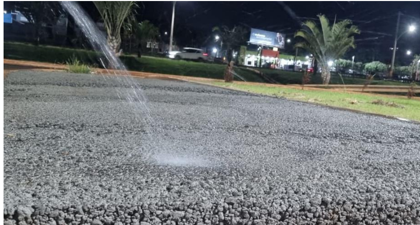
Figure 4 - Pervious concrete test track with construction waste. Source: Author himself.
